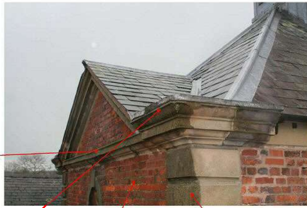
In periods of persistent rainfall, cement mortar can prevent water evaporating at the surface of the joint, resulting in saturation of the wall
